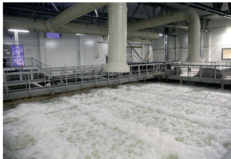
Submerged aeration system for degassing in RAS at Mowi facility in Nordheim. Photo: Kevin Stiller/Nofima
